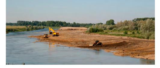
Existing gravel pits were integrated into the river system by lowering the banks.
