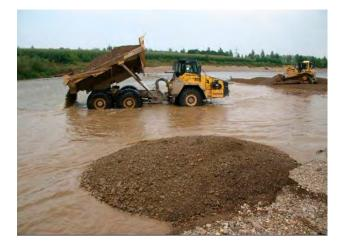
Where possible, gravel was also added to the incised river bed. The gravel augmentation from the Flemish banks amounts some 400,000m<sup>3</sup> of gravel.
